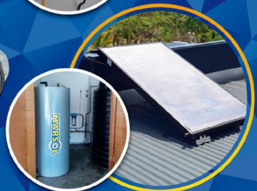
CONVERSION OF ELECTRIC BOILER TO SOLAR WATERHEATER
