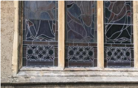
Same window after restoration
