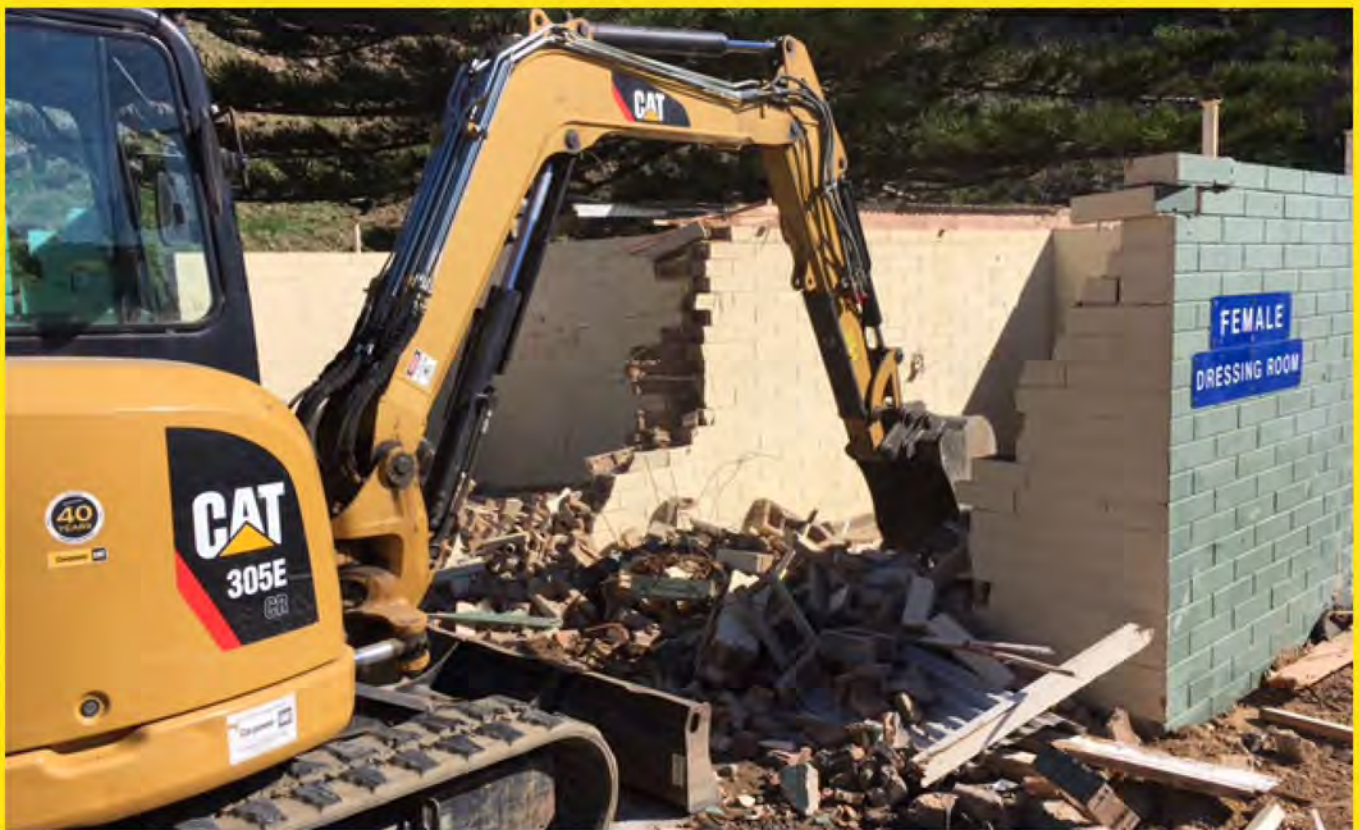
Image: Second Valley Toilet Block Demolition
