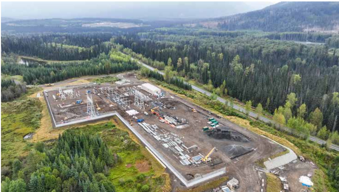
Recent milestones of the KSM project include construction of the Treaty Creek Switching Station to deliver clean hydroelectric power to the project.
