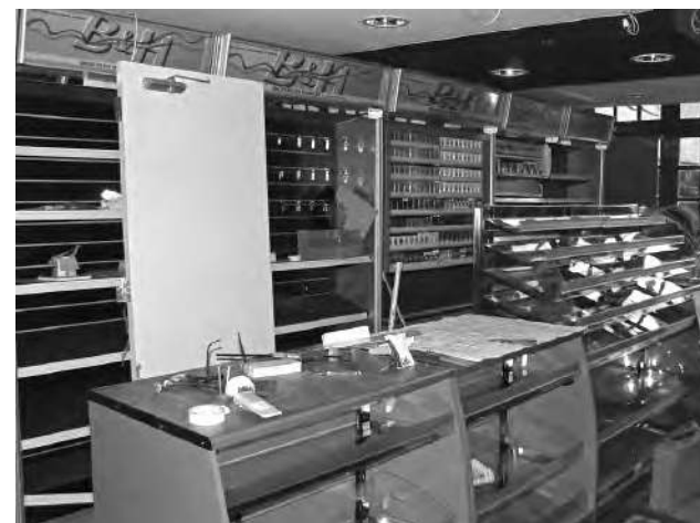
Work on the new shop is progressing fast. Photo: Hugh O' Brien
