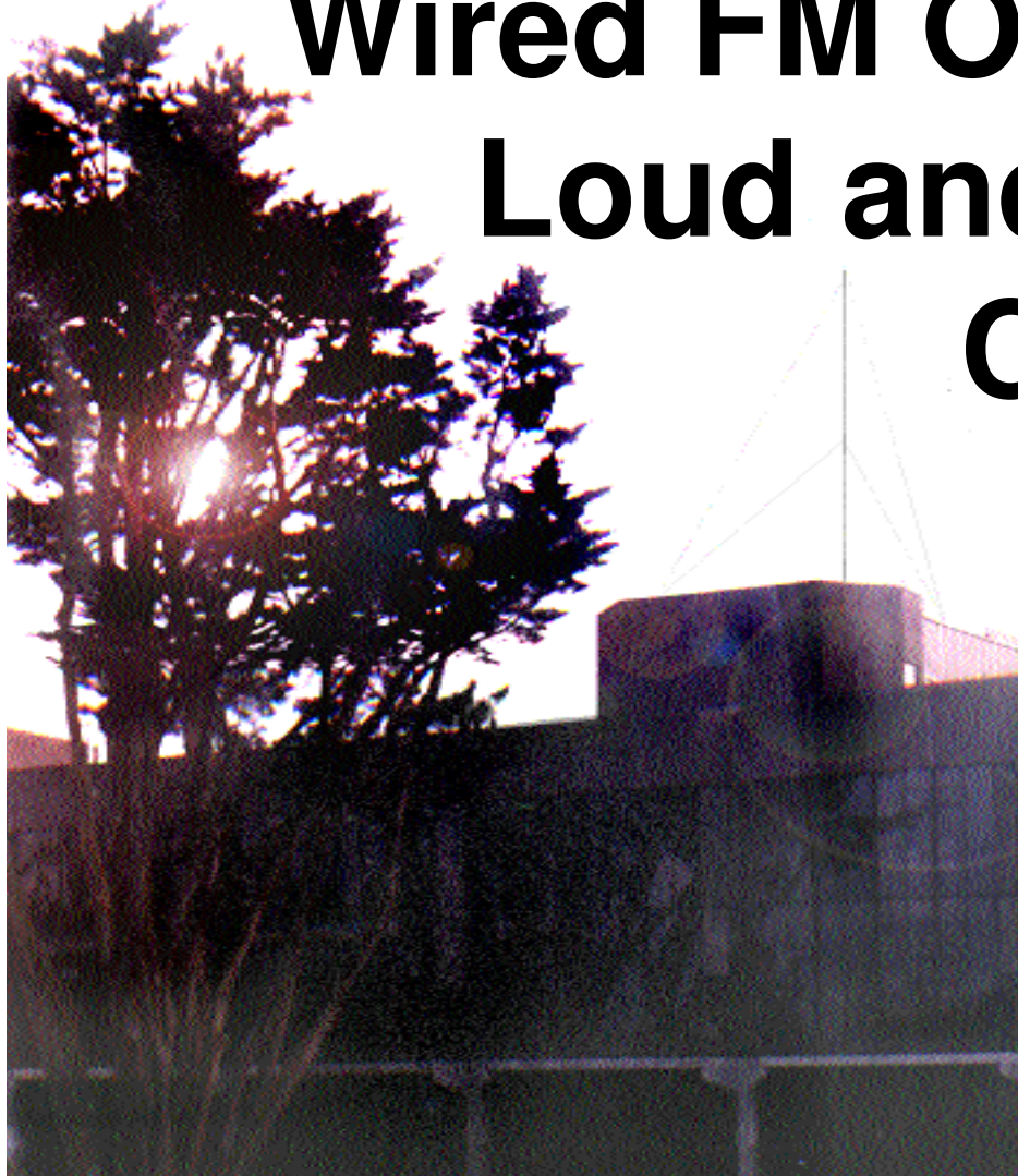
The new transmitter for Castletroy situated on the roof of the main building
