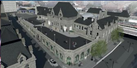
£34m Rail Station upgrades
