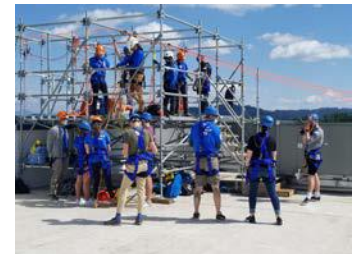
Scaffolding on the roof
