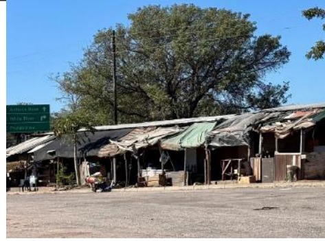
Plastic View after the fire (far left), more shacks near Jonkmanspruit (middle) and shacks opposite Build It.
