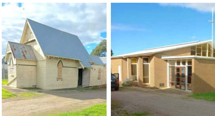
Moriac Uniting Church A new church was built alongside the original in 1971
