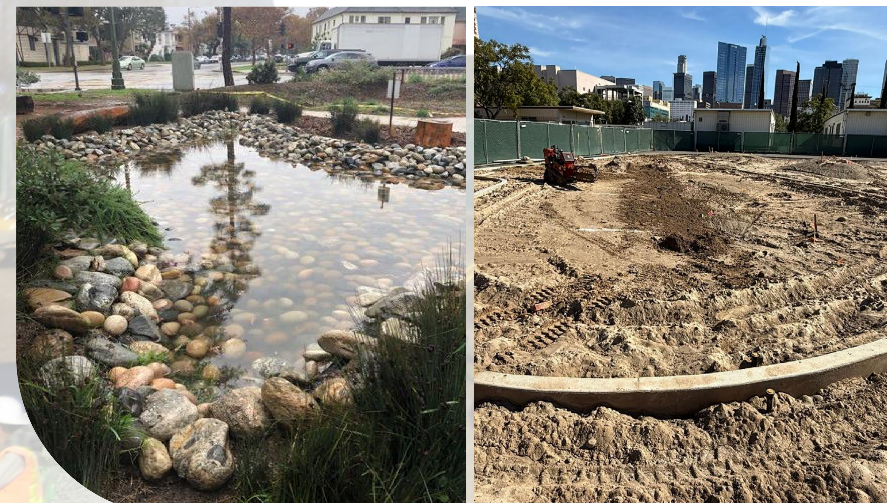
(bottom-left) Infiltration swale at Carthay Environmental Magnet; (bottom-right) Bioswale construction at Esperanza Elementary
