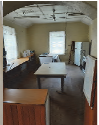
The kitchen will be fully replaced
