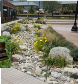
Infiltratlon Swale
