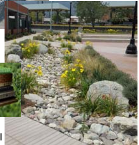
Infiltration Swale
