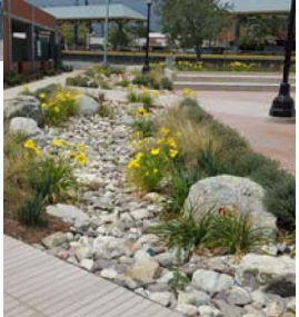
Infiltration Swale
