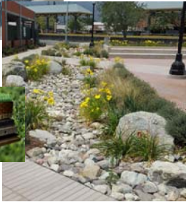
Infiltration Swale
