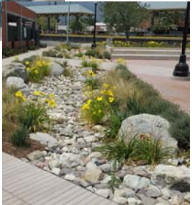
Infiltration Swale
