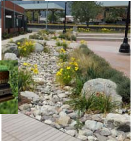
Infiltration Swale
