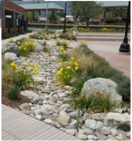
Infiltration Swale
