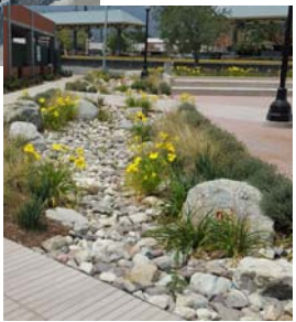
Infiltration Swale
