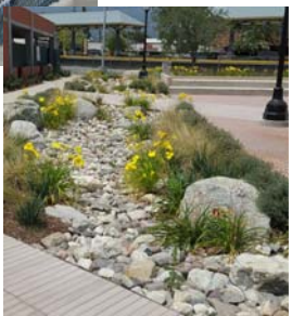
Infiltration Swale
