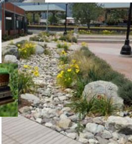
Infiltration Swale
