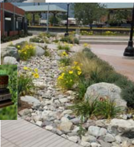
Infiltration Swale
