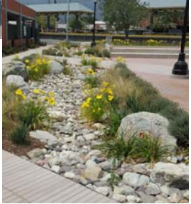
Infiltration Swale
