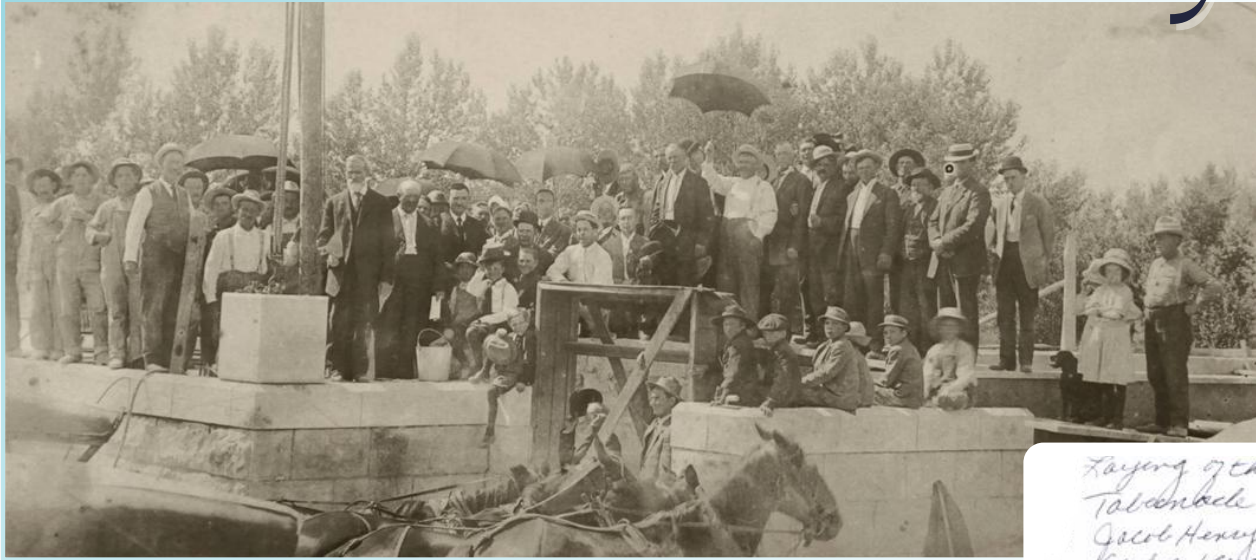
Groundbreaking of the Rexburg Tabernacle
