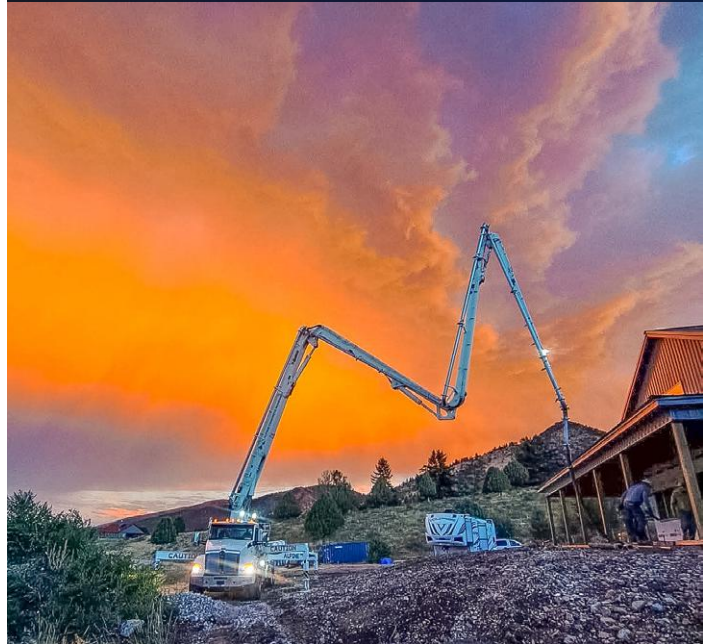
Submitted by ALPINE CONCRETE PUMPING Morgan, UT
