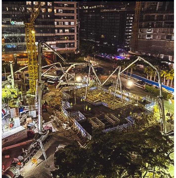
Submitted by FLORIDA CONCRETE UNLIMITED Miami, FL
