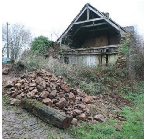
The demolition of the ruin will have to wait
