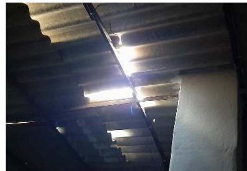
Damages at Samarth
