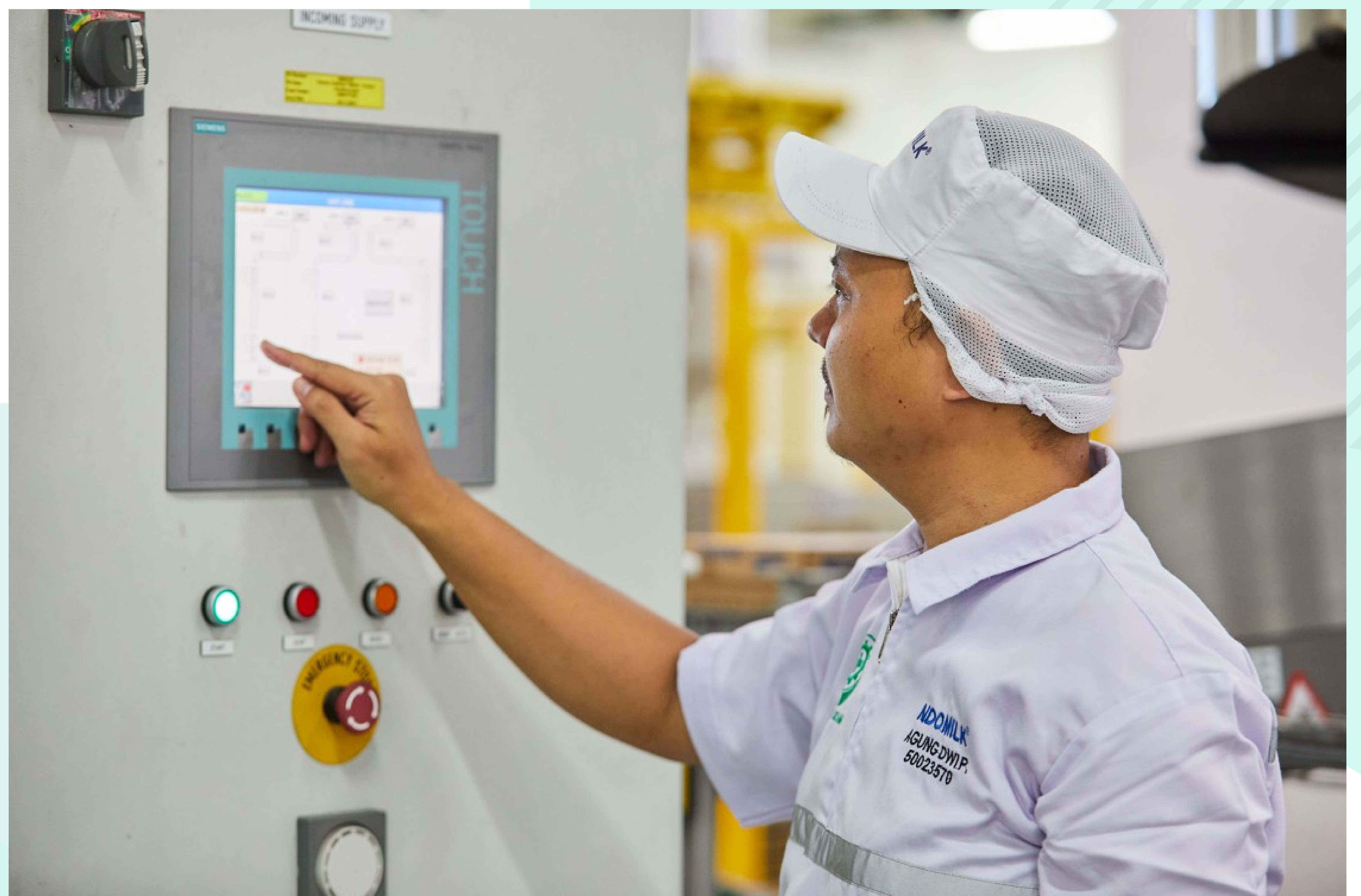
Indolakto makes use of Siemens' flagship automation system including HMI (photo: Ralf Baumgarten)
