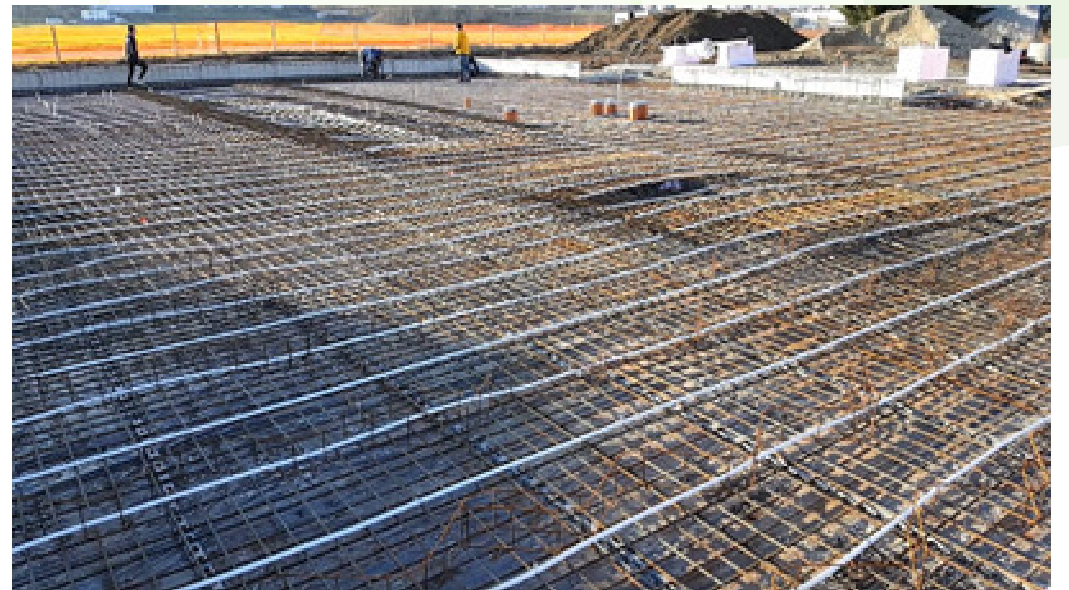
Electric heating wires will activate the concrete foundation of the building in the future.
