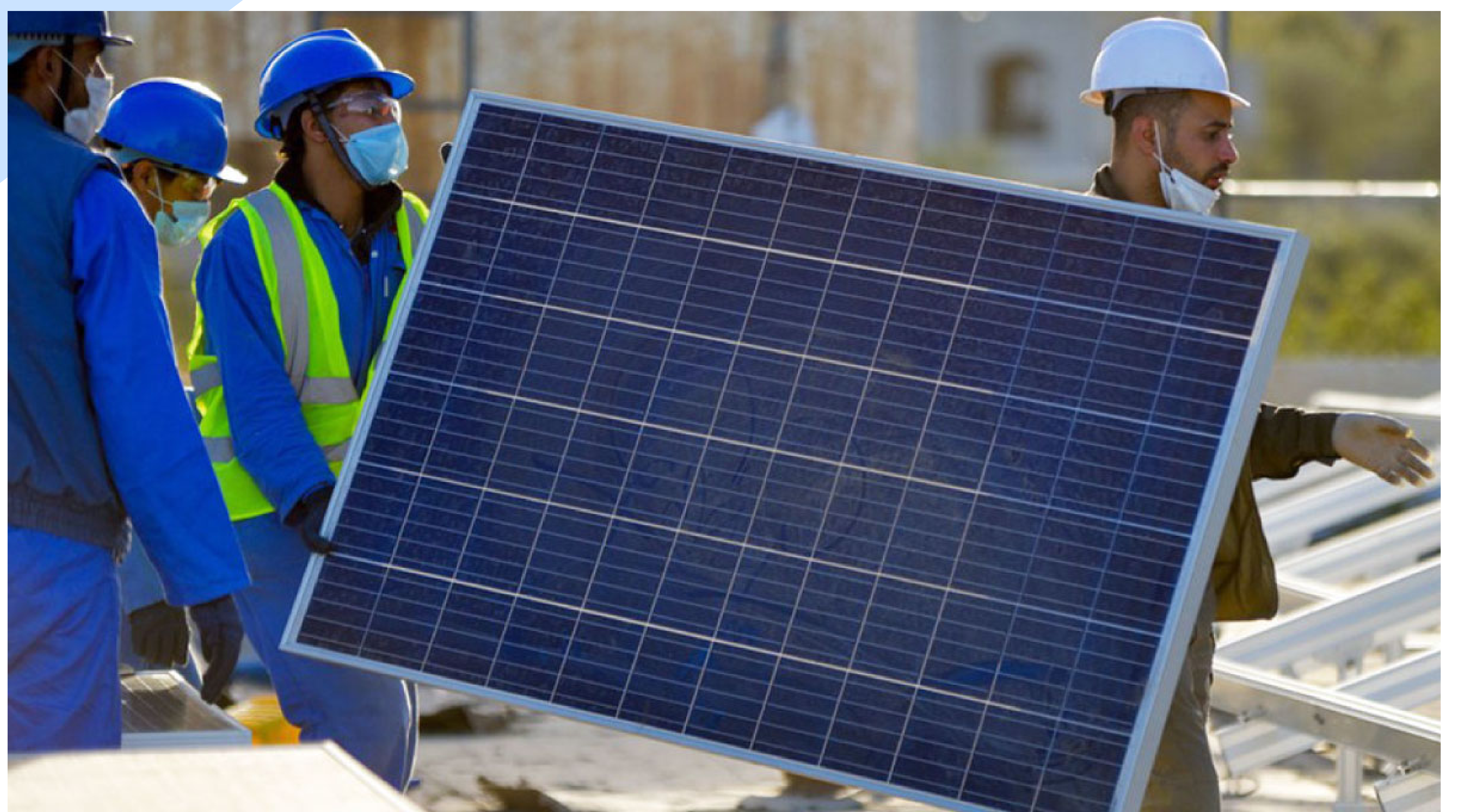
Workers install solar panels for a hospital in Yemen. / © UNDP Yemen
