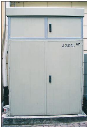
The Cabinet after extension
