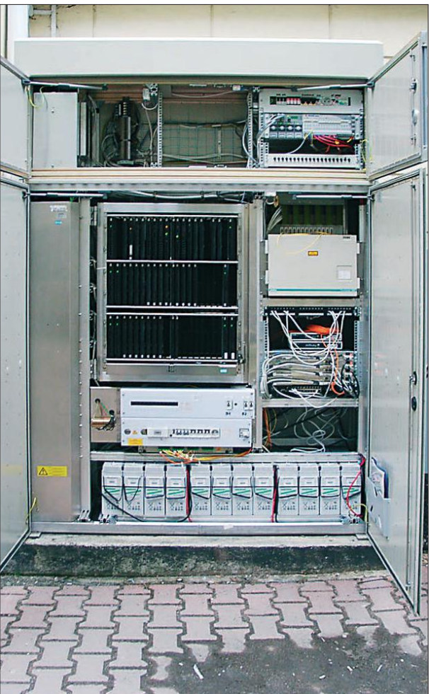
The cabinet after extension
