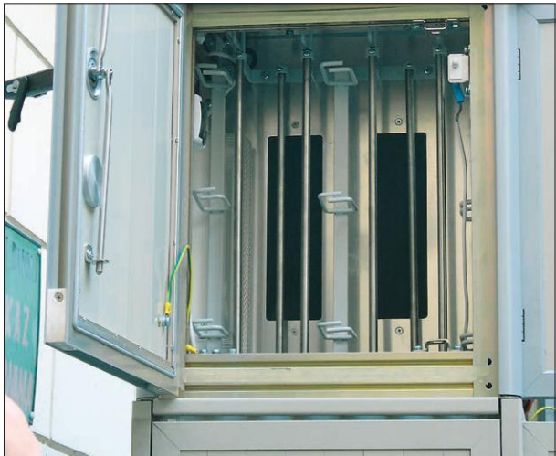
The cabinet after extension
