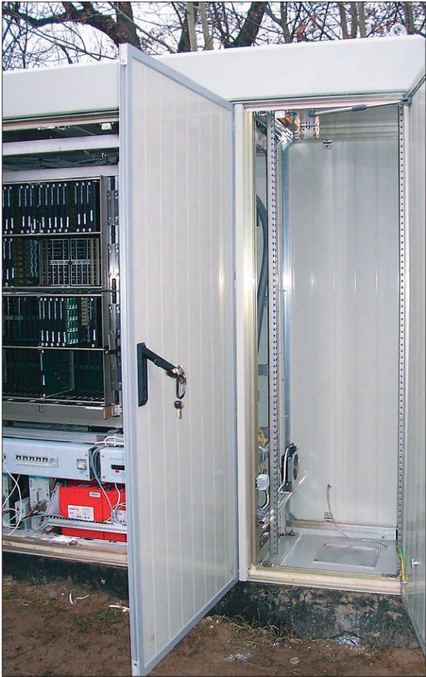
The cabinet after extension
