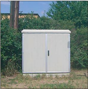
Cabinet before extension
