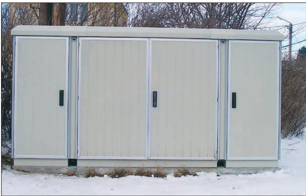
The cabinet after extension
