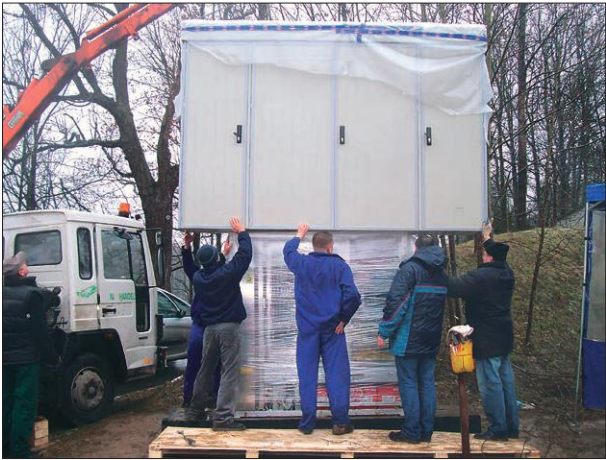
Cabinet during extension
