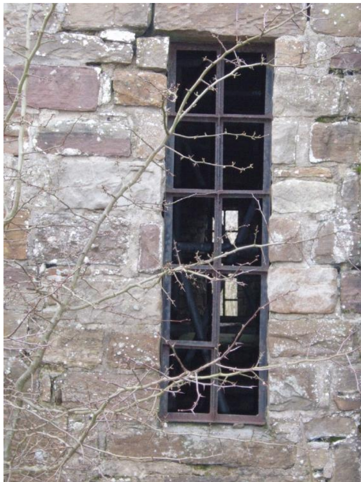
An iron window frame in the tower
