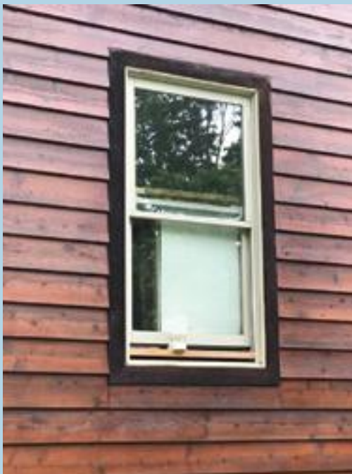
The outside view of the hive box. The matte board is dark inside but white outside. It slides between the hive box and the window of the bedroom. The bottom gap is the space between the floor/landing board and the window sill. The next gap is the entrance for the bees.
