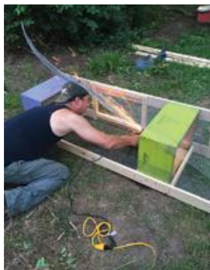
Grinding down the edges.
