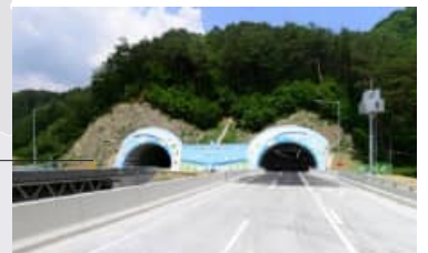
Inje Yangyang Tunnel
