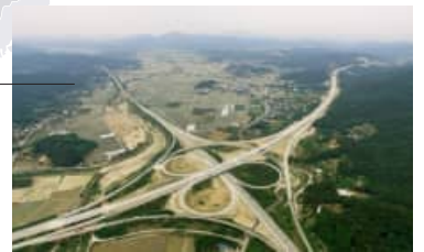
Sangju Yeongcheon Expressway
