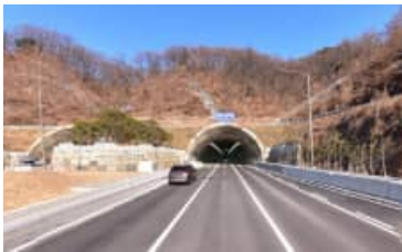
Yongin Branch Tunnel
