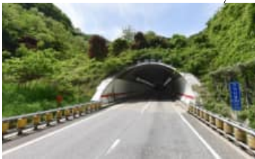
23 locations including Godeok Tunnel
