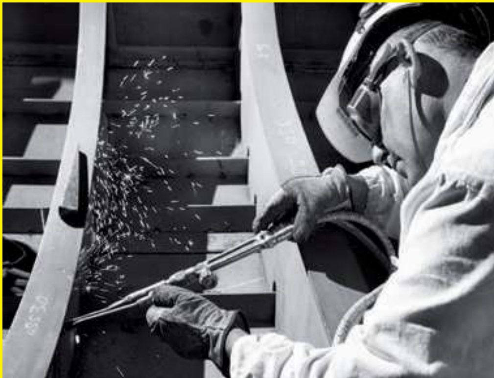
Craftspeople express their artistry once the hull is built, with the structural work, fitting out, and installation of onboard systems
