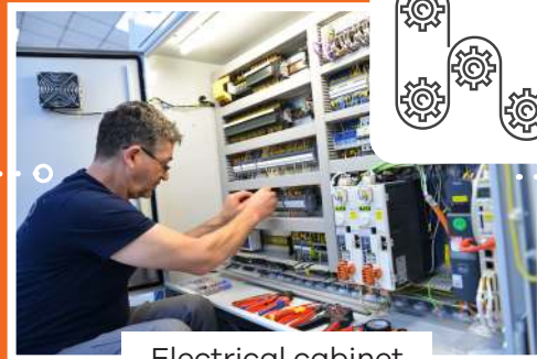
Electrical cabinet assembly
