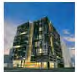
Guilfoyle Apartments South Melbourne
