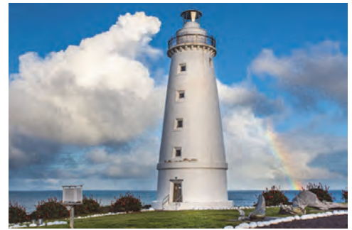
Cape Willoughby Lighthouse (source: DEWNR)
