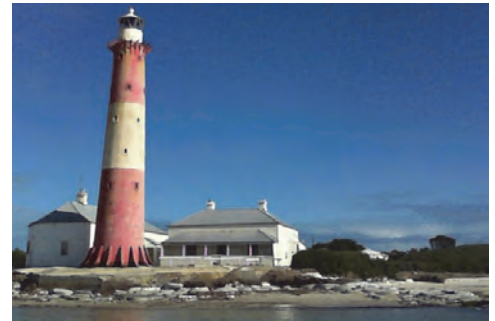
Troubridge-Island-Lighthouse (source: DEWNR)
