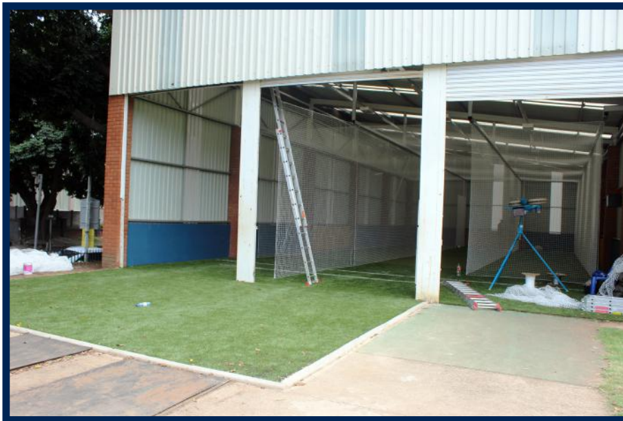
High Performance Cricket Facilities Upgrade
