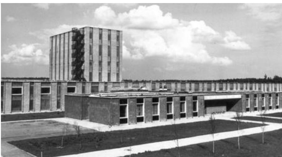
1984 – Võru Bread Factory. Architect: Ado Eigi
