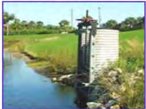
Operable Discharge Control Structure
