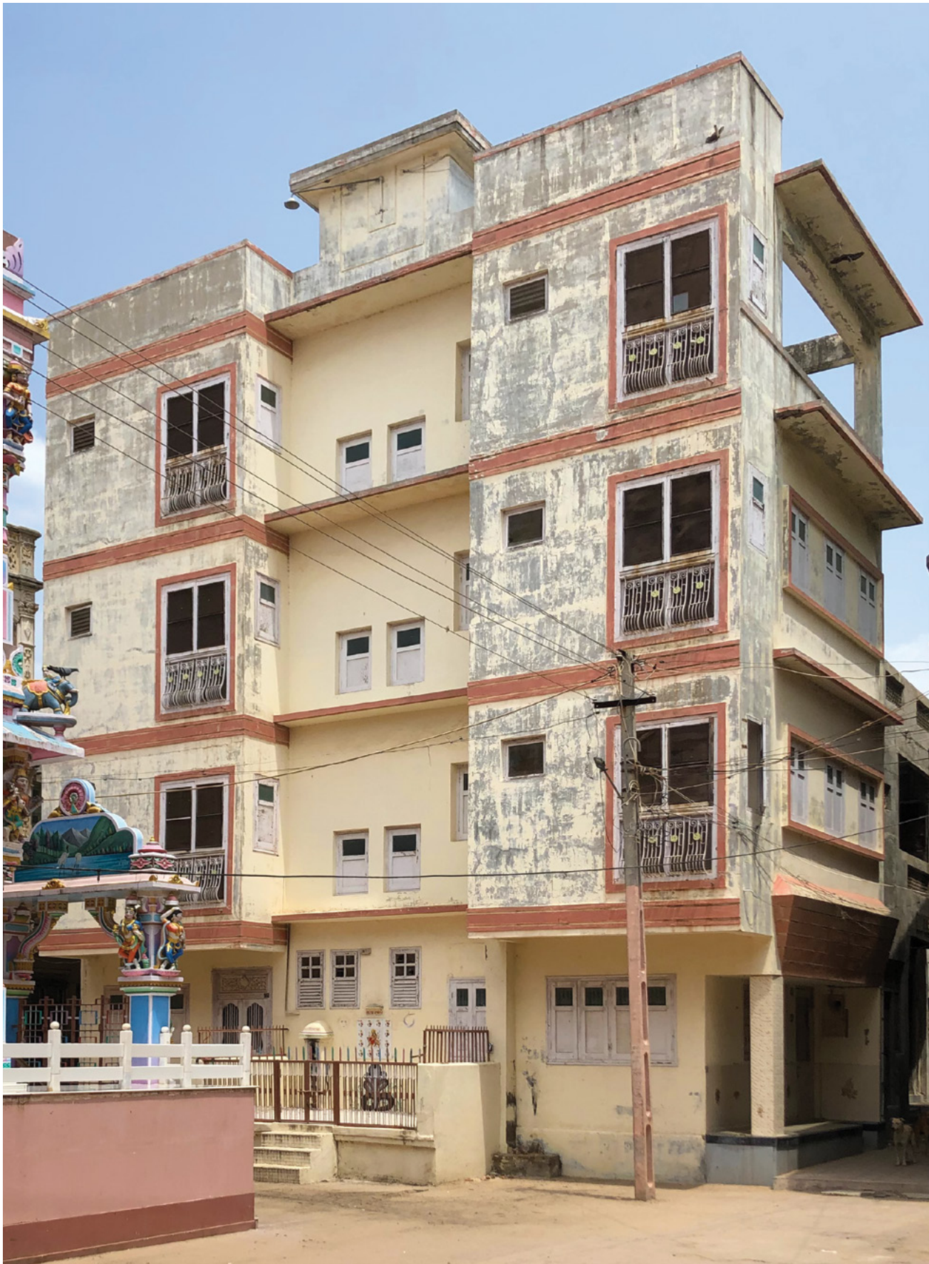
PANNALAL MAFATAL MANIAR'S HOUSE IN CHODHRI NI SHERI, PATAN. IT WAS RECONSTRUCTED IN 1974
