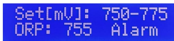
Figure 6 - Main Menu with an Active Alarm
