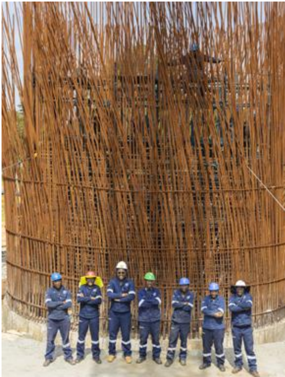
To address the seismic risk, installing the reinforcing steel was especially demanding, with more than 210 kilograms of rebar required per cubic metre
