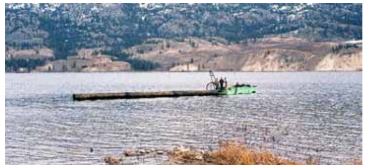
New intake pipe being float/towed into place.
