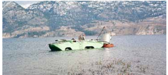
New intake on its way to the bottom.
