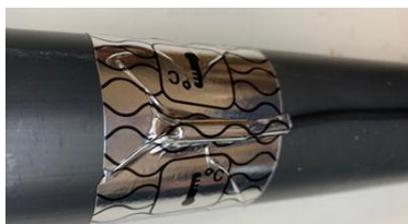
Figure 6 – Temperature Probe Installation
