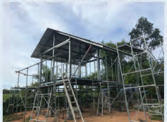
House build Day 3
