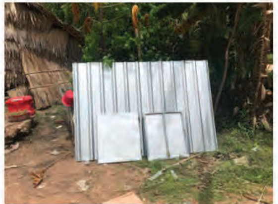
House build Day 2
