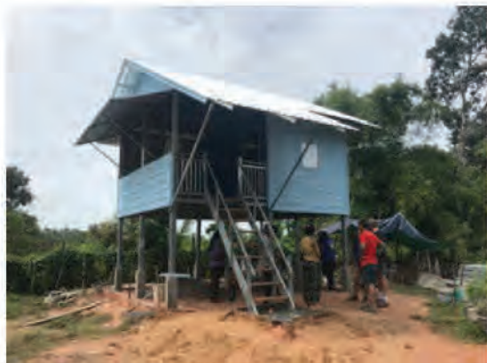
The finished house!
