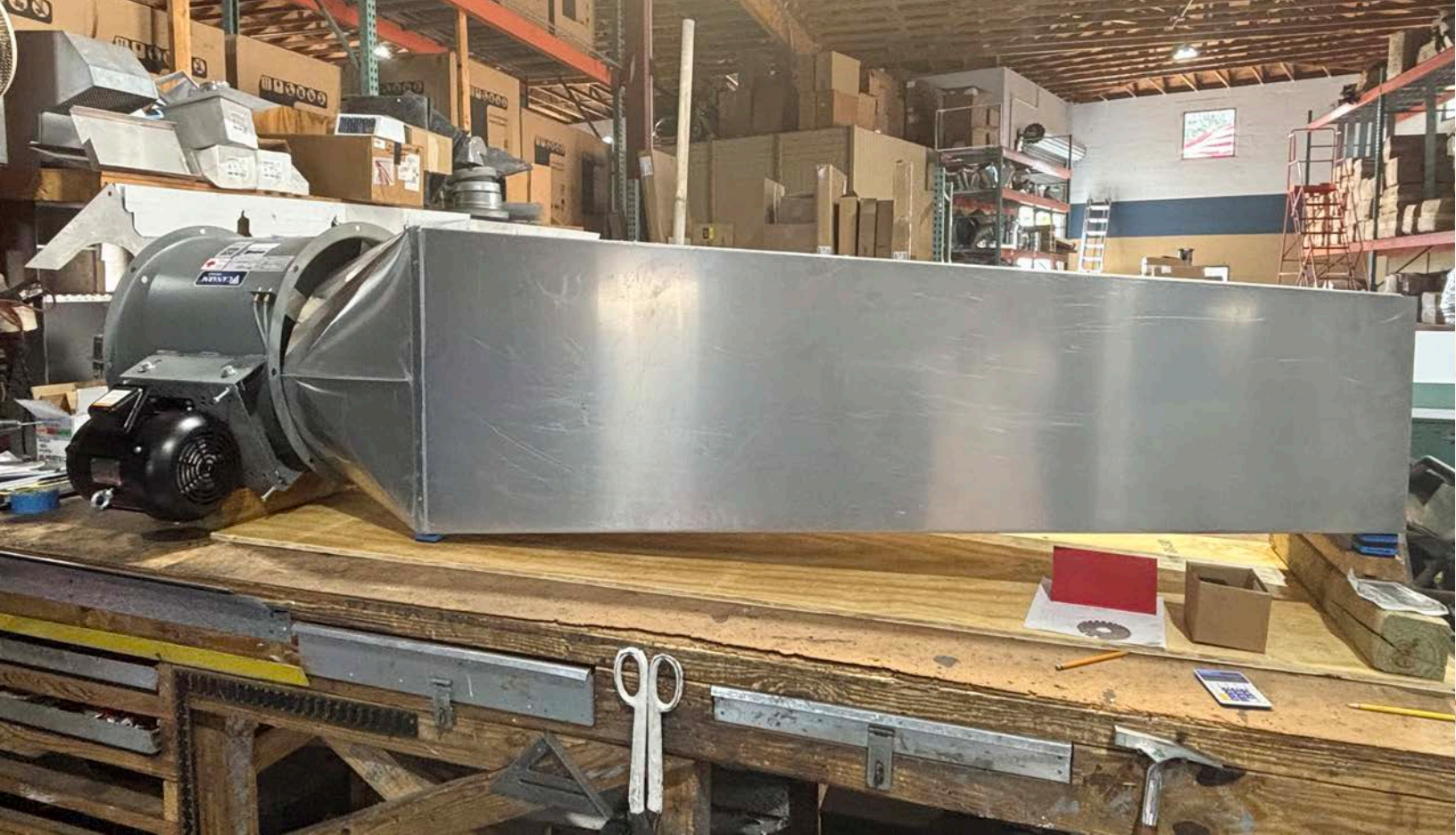
Above: From foam board to properly rated aluminum, the idea becomes a reality. Below: Sourcing the industrial fan was crucial to the project's forward momentum.
