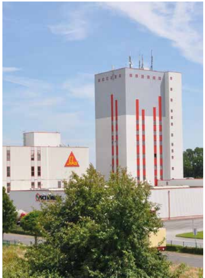
The PILOT:MES Manufacturing Execution System from FELTEN at Sika's Rosendahl site guarantees that the filling process is in continuous flow. (Source: Sika)
