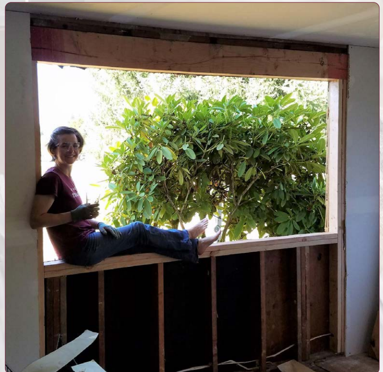
This is a photo of our '70s ranch house remodel, which we started in 2018 and took down to studs. We had just expanded this bedroom window and added a new header (the beam at the top).
