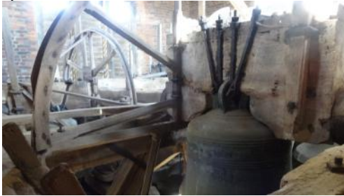
Dedham Church bell chamber showing the remains of the full wheels.
