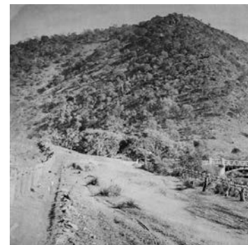
Picture: The Gorge, Yankalilla, 1871, depicting vegetation on the coastal cliffs, near where present-day Main South Road crosses the Yankalilla River.
