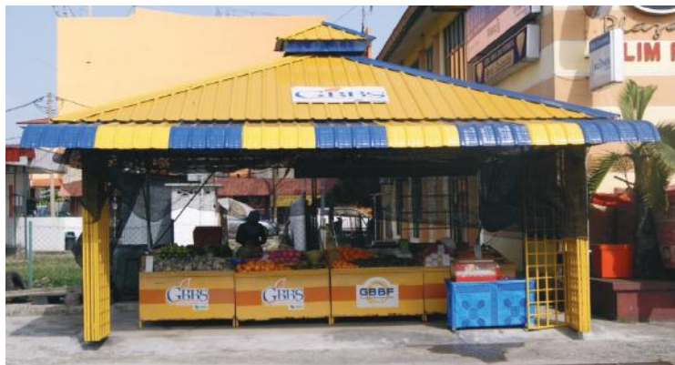
GBBS Separa Kekal (Berbumbung metal deck bersaiz 20' x 20') GBBS Konsep Metal Deck. Lokasi di Tanjung Malim, Perak Semi Permanent GBBS (metal deck cover 20' x 20') Located at Tanjung Malim, Perak
