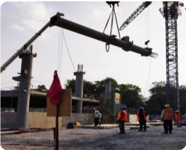
February 5 (Day 5) : Ground Floor Columns and Erection
