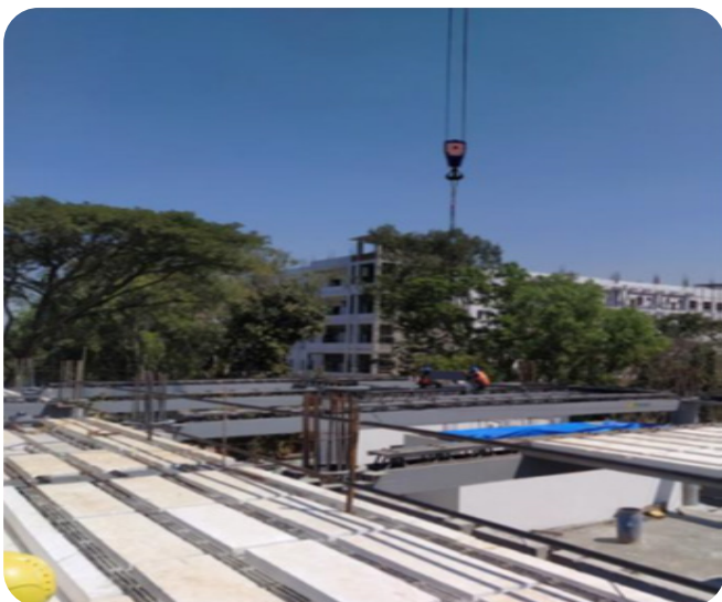
February 6 (Day 6): Beams erection
