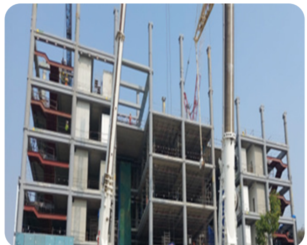
February 25 to 27: Sixth Floor Beams and Slabs erected.
