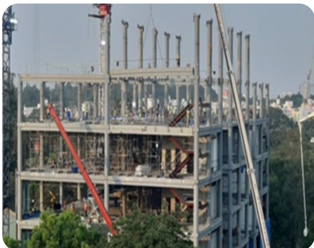
February 23 & 24: Fifth Floor Beams & Slabs Erected.
