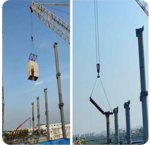
February 19: Prefabricated prefinished lift pods & prefabricated stair case erected.
