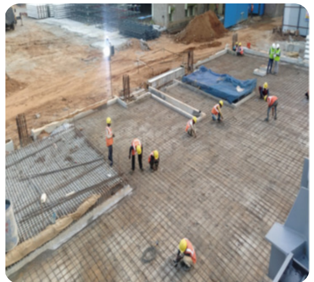
February 1st (Day 1) Grade Slab Reinforcement
