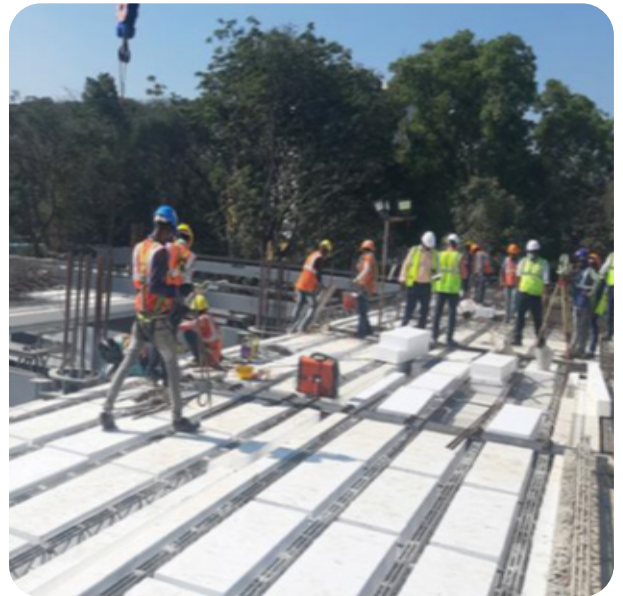
February 10 & 11: Second Floor Slab and erection of beams
