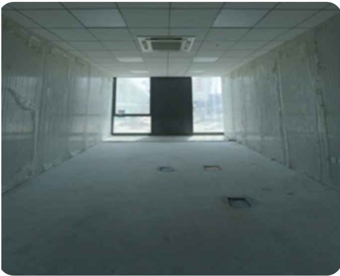
February 28: Prefinished modular walls are installed in the first floor on false flooring system.
