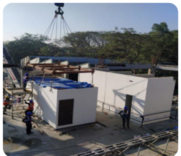
February 7 (Day 7): Positioning of prefabricated prefinished toilet pods
