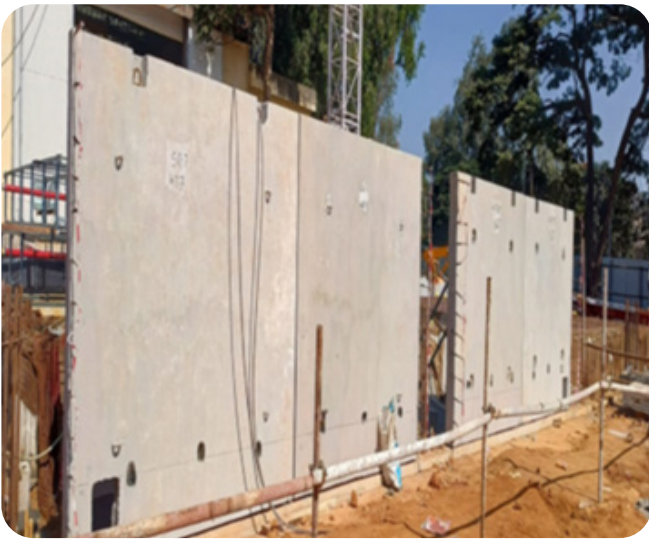
February 3 (Day 3): 2D Precast RC walls on GF
