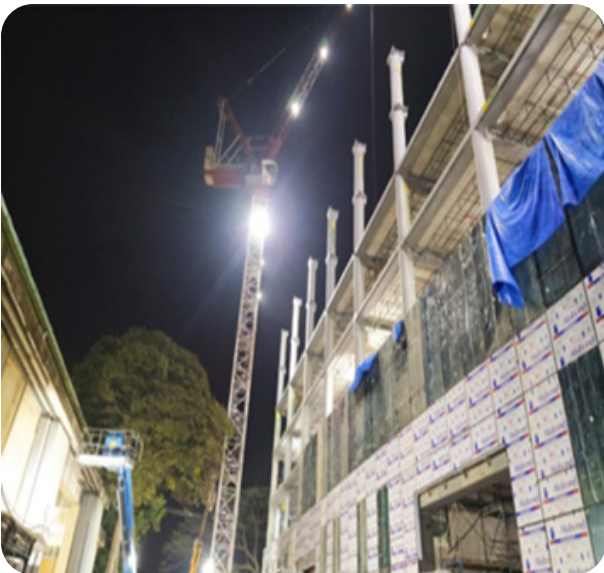
February 20 & 21: Unitized structural glazing system installation at ground floor and first floor
