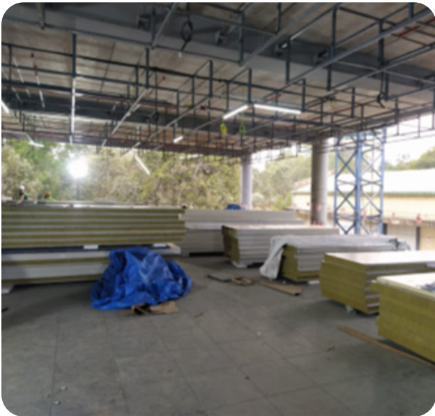
February 8 & 9 (Day 8 & 9):Interior wall panels and other interior elements stacked.
