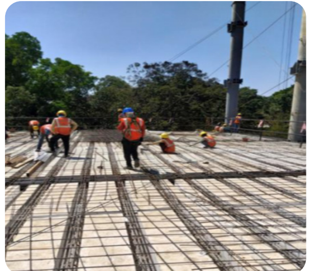
February 6 (Day 6) : First Floor Slab
