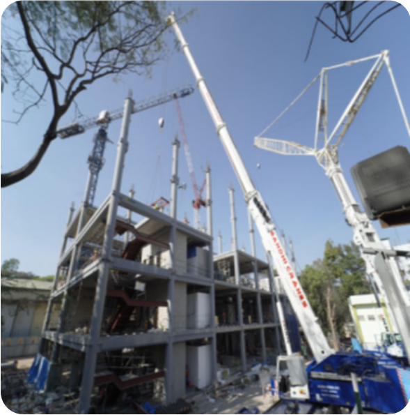
February 18: Third Floor Structural Elements are erected
