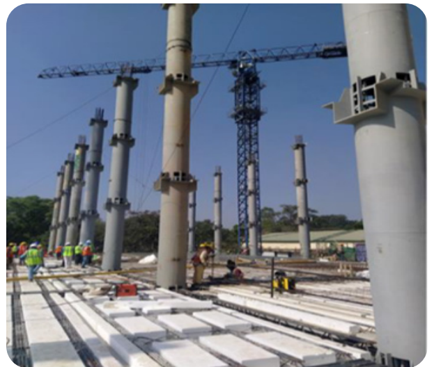
February 12 & 13: Structural Column Splice at Second Floor Level
