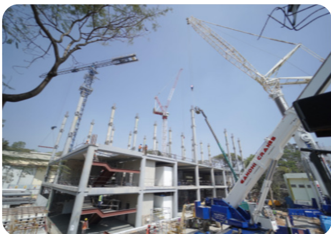
February 14 & 15: Second to Fourth Floor Columns Erected
