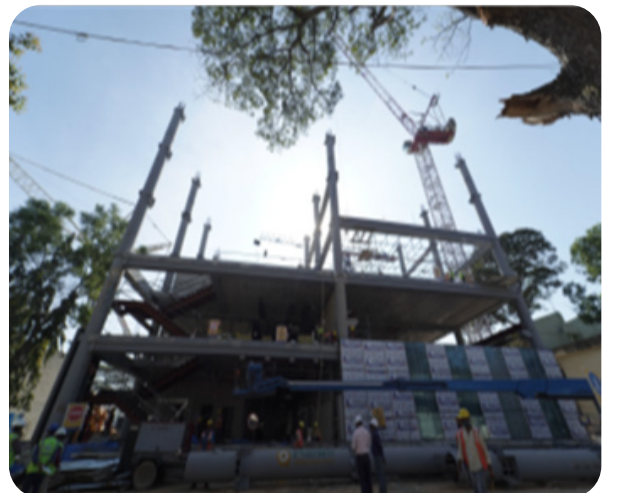
February 16 & 17: Second Floor prefabricated cradle is lowered,Second Floor Structural Elements & toilet pods on third floor erected
