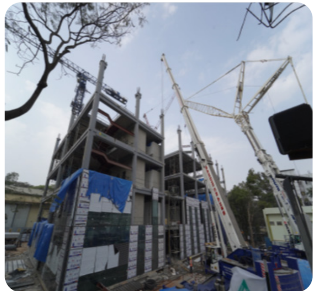
February 22: Fourth Floor Structural Elements Erected.
