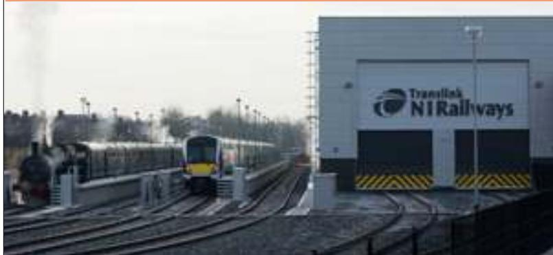
The works included the construction of a new train care maintenance facility on Translink's existing site in Adelaide, Belfast. The project comprised of a new train maintenance building, accommodation buildings and offices, refurbishment of an existing operations building and, infrastructure works including new HV distribution system, new train wash facility, fuelling apron and oil storage facilities.
