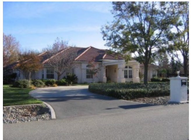
Single-family residential home. Photo courtesy of the Butte County Department of Development Services.
