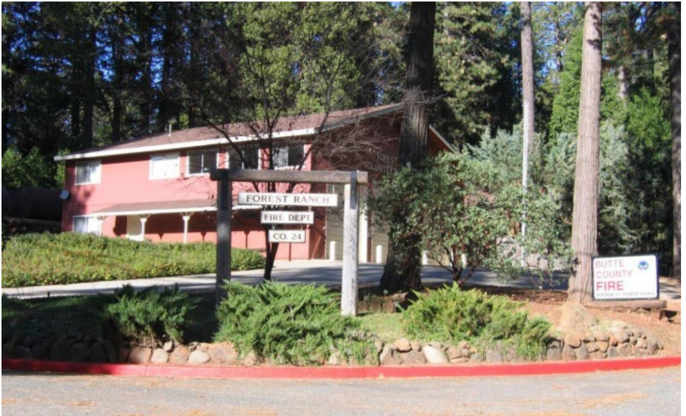
Forest Ranch Fire Department. Photo courtesy of the Butte County Department of Development Services.
