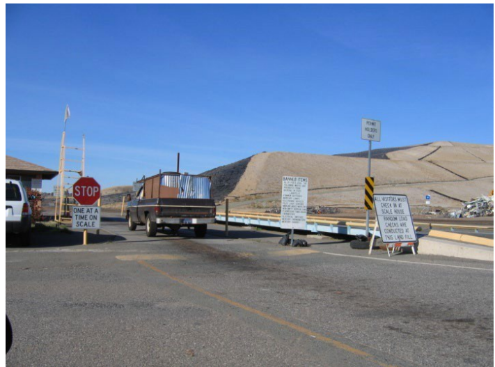
Neal Road Recycling and Waste Facility. Photo courtesy of the Butte County Department of Development Services.
