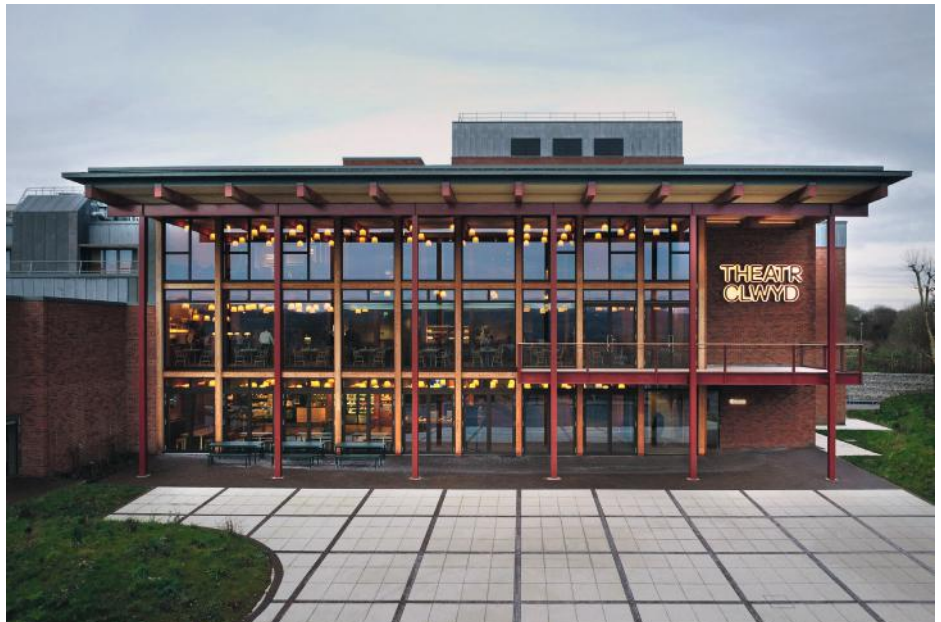
Below: The extension is glulam-framed, with external steel posts for weather resilience.
