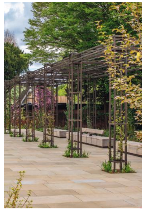
Above: The pergola utilises steels salvaged from a greenhouse previously on the site.
