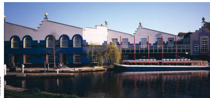
Right Rear (canal-side) view of the TV-am studios in Camden, London, 1981.
