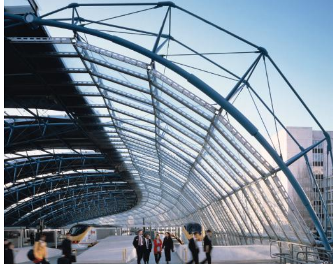
Right At Waterloo, the curving site is dealt with by adjustable tubular steel portal frames and lapped sheets of glass.
