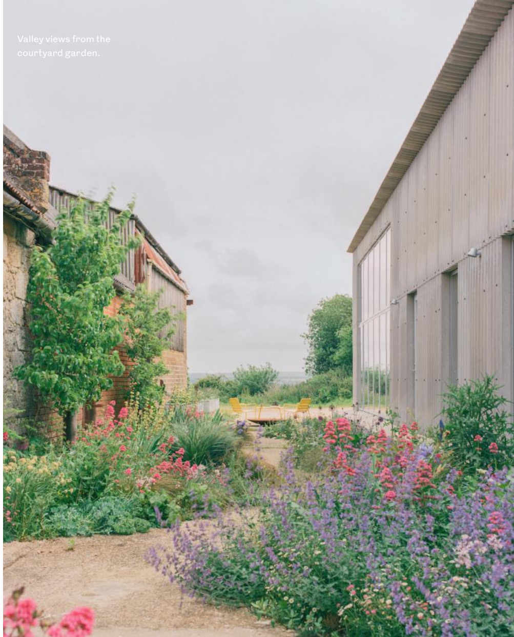
A glazed screen on the southeast corner is part-shaded by barns opposite.
