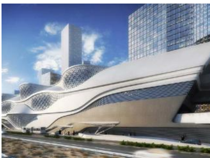
KAFD Metro Station, Saudi Arabia
